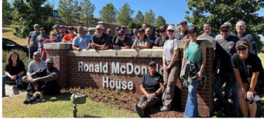
▲ Our UNBRIDLED ESP Systems team came together to improve lives recently – building a new fence and improving landscaping at the Ronald McDonald House in Tulsa, OK.
